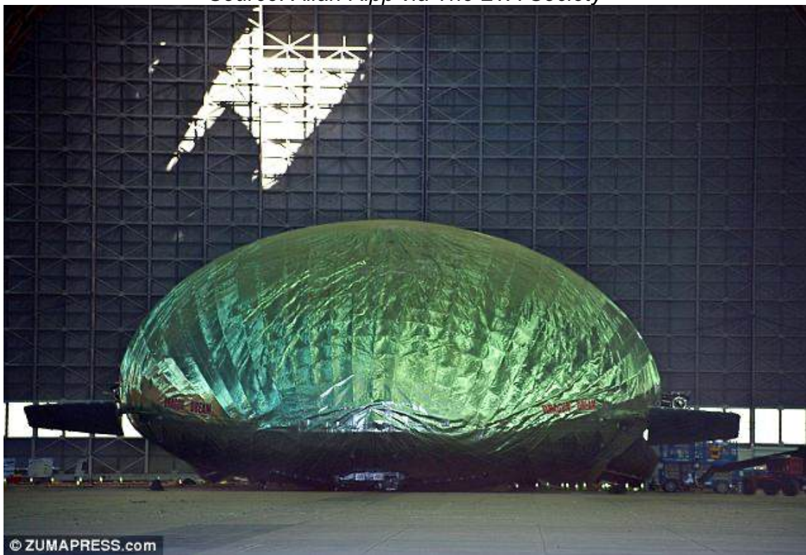
The undamaged front part of the ML806 Dragon Dream after the roof collapse. Source: ZUMAPRESS via Daily Mail
