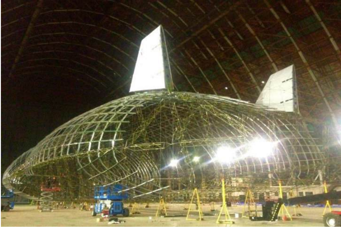
The ML806 Dragon Dream's assembled lightweight, rigid aeroshell frame is installed around the internal main frame.
